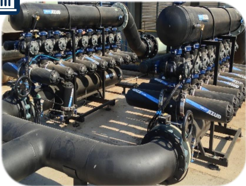
2 x AZUD HELIX AUTOMATIC 4DCL9 450 m 3 /h | 100 μm | Chile AGBAR Santiago WWTP
