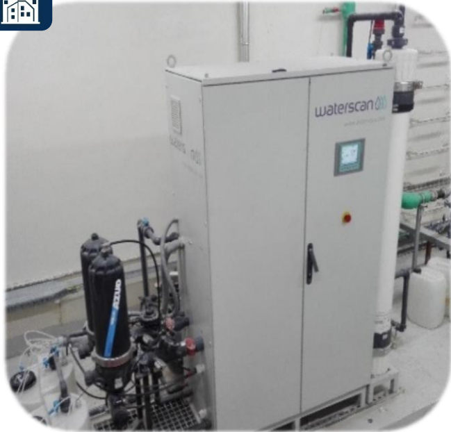
1 x AZUD HELIX AUTOMATIC 201 AA 3 m 3 /h | 100 μm | Qatar Education city Premier Inn Hotel
