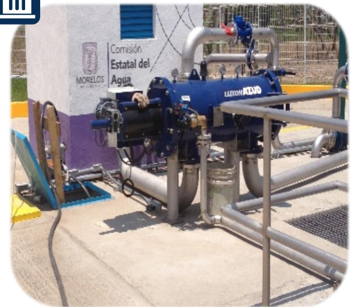
1 x AZUD LUXON LXE 5400 S/6 50 m 3 /h | 50 μm | México Temoac Morelos WWTP
