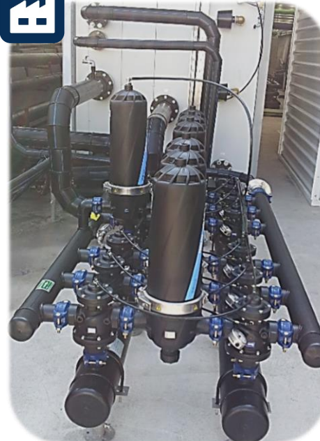
2 x AZUD HELIX AUTOMATIC FT205 AA 150 m 3 /h | 100 μm | Mexico VOLKSWAGEN- Puebla
