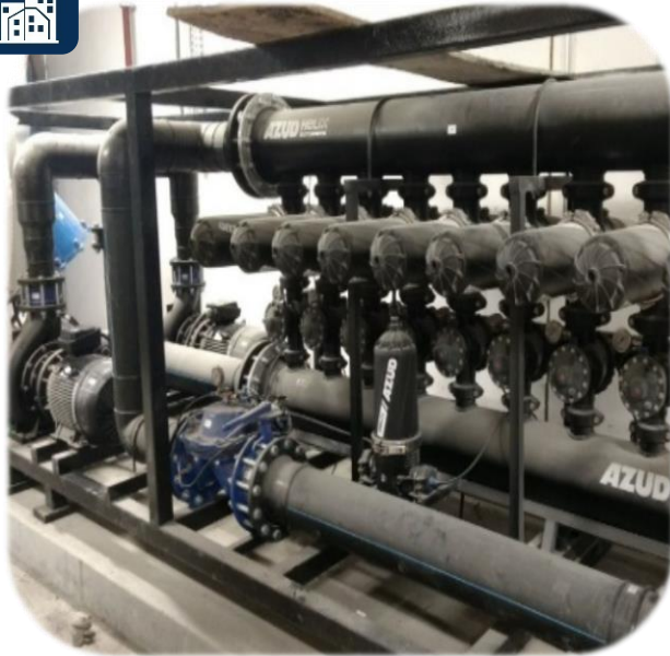
1 x AZUD HELIX AUTOMATIC FES 4DCL9 250 m 3 /h | 50 µm | Dubai Apartamentos Emirates Hills
