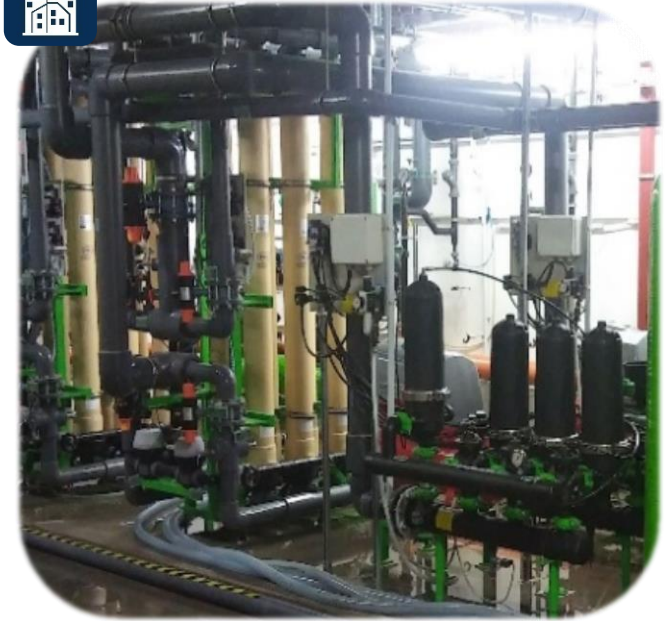
1 x AZUD HELIX AUTOMATIC FT203 AA 60 m 3 /h | 50 μm | Alemania Holmes-Place fitness center spa
