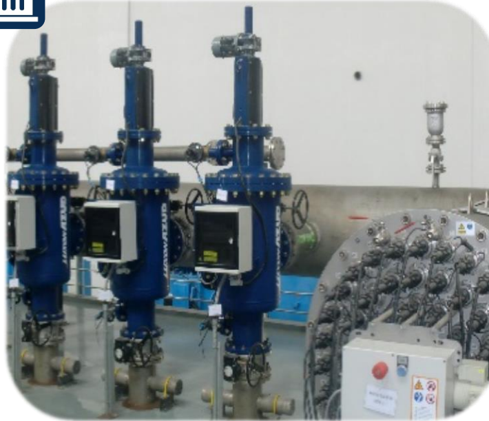
8 x AZUD LUXON LDB 8000 S/8 1.600 m 3 /h | 25 μm | China Shanghai Disney resort
